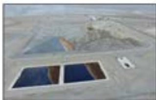
Figure 1: Leachate collection in be'ah landfill
