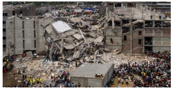
Figure 6 Eight storey commercial building named Rana Plaza, collapsed Bangladesh (Source: Wikipedia 24 April 2013).
