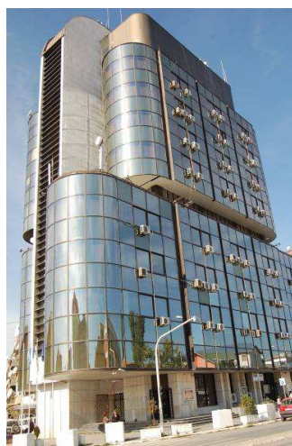
Fig 2 View of the HQ building at Prishtina, Kosovo
